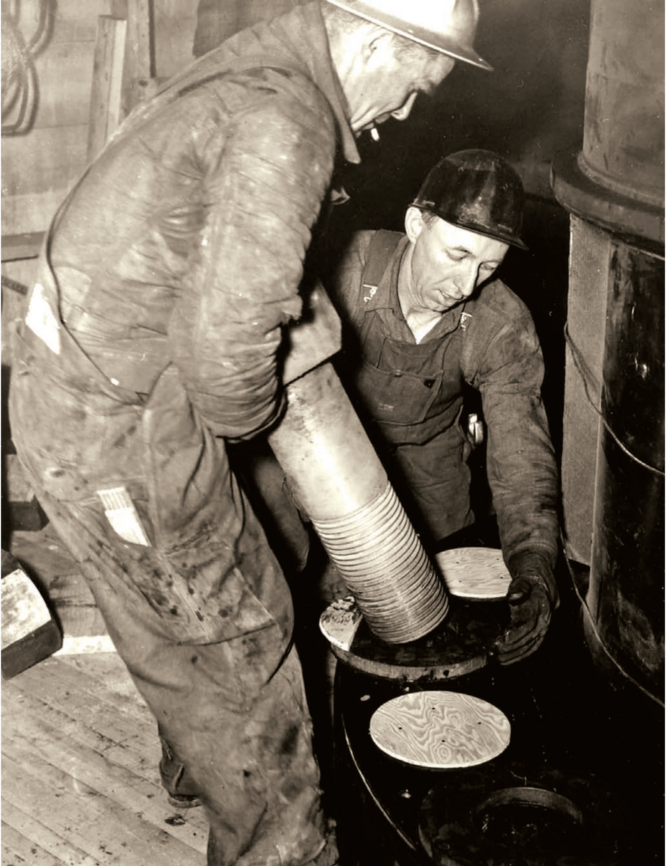
AMOS "TEX" WOOD, STANDING, HELPS POSITION ONE OF THE 120-POUND BOLTS WHICH HOLD THE ROTOR SHAFTS TOGETHER. GRAND COULEE DAM, FEBRUARY 11, 1941.
