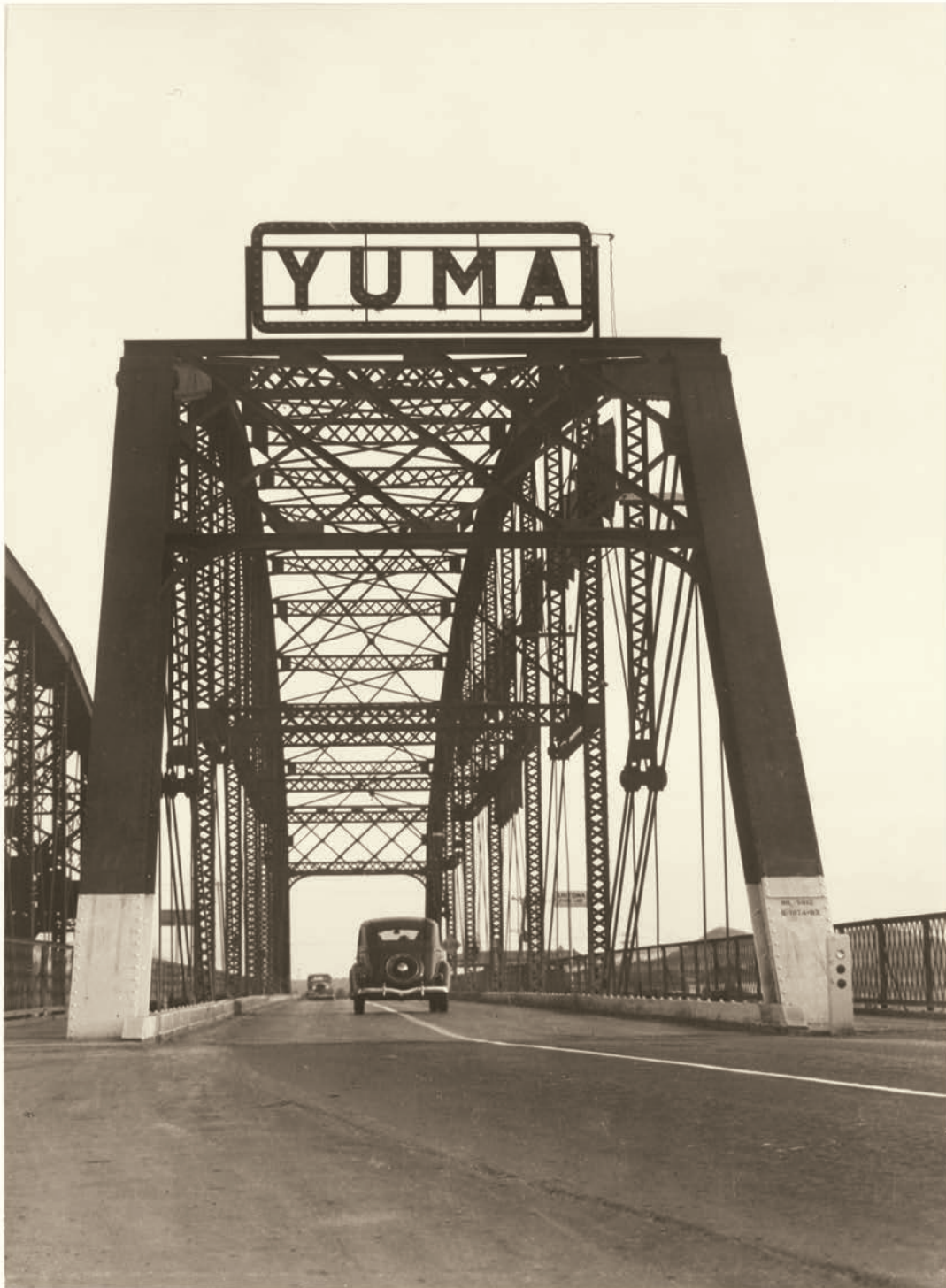
Franklin D. Roosevelt 1935 Over this bridge drought refugees are crossing the Colorado River into California, U.S. 80
