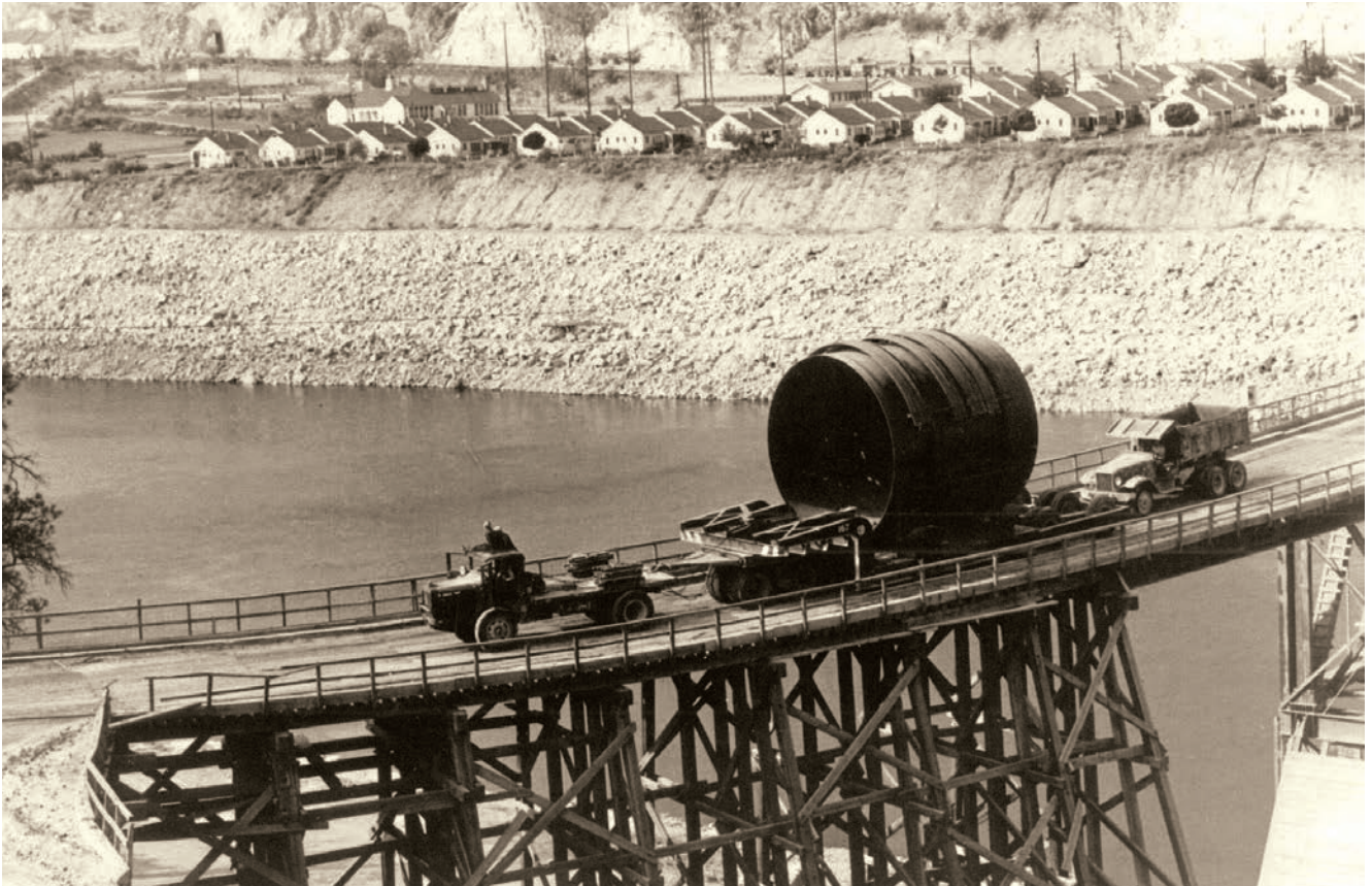
MOVING A PENSTOCK SECTION AT GRAND COULEE DAM, CIRCA 1941.
