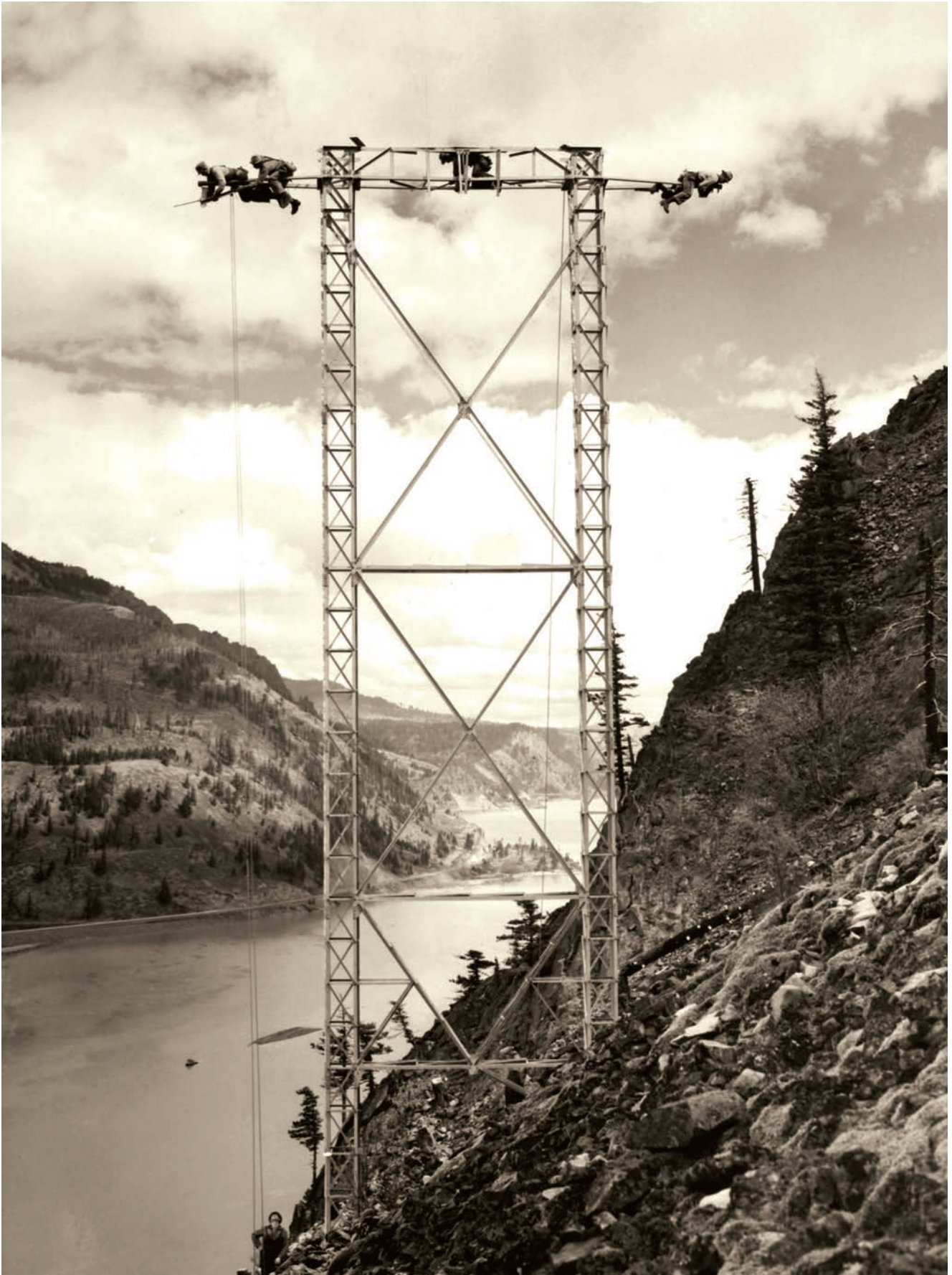
LINE CONSTRUCTION AT THE DALLES, 1941.
