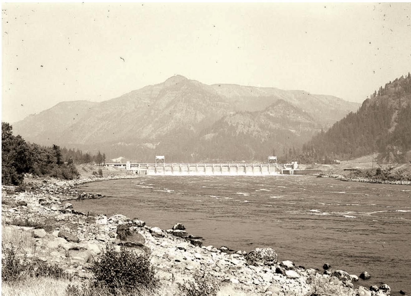
BONNEVILLE DAM DOWNSTREAM, 1940.
